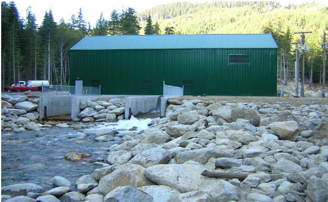
Figure 9: Powerhouse at Furry Creek.
